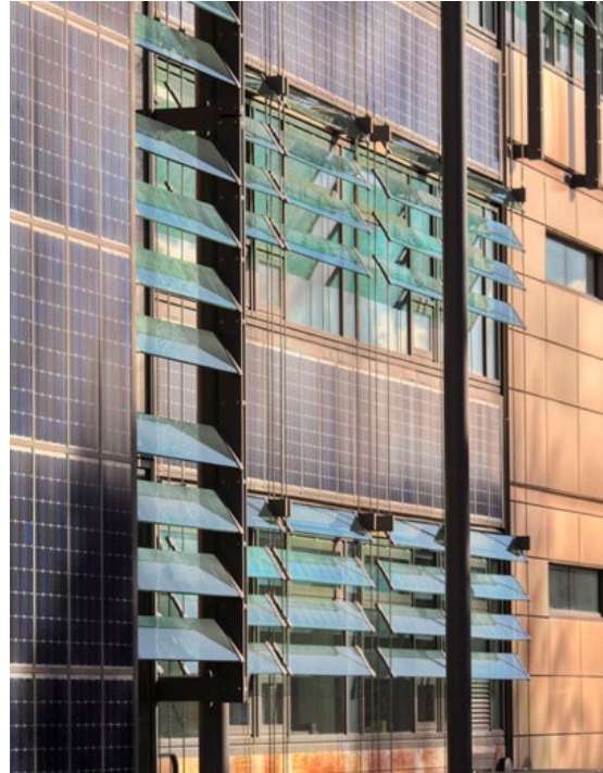
Building Integrated PV
